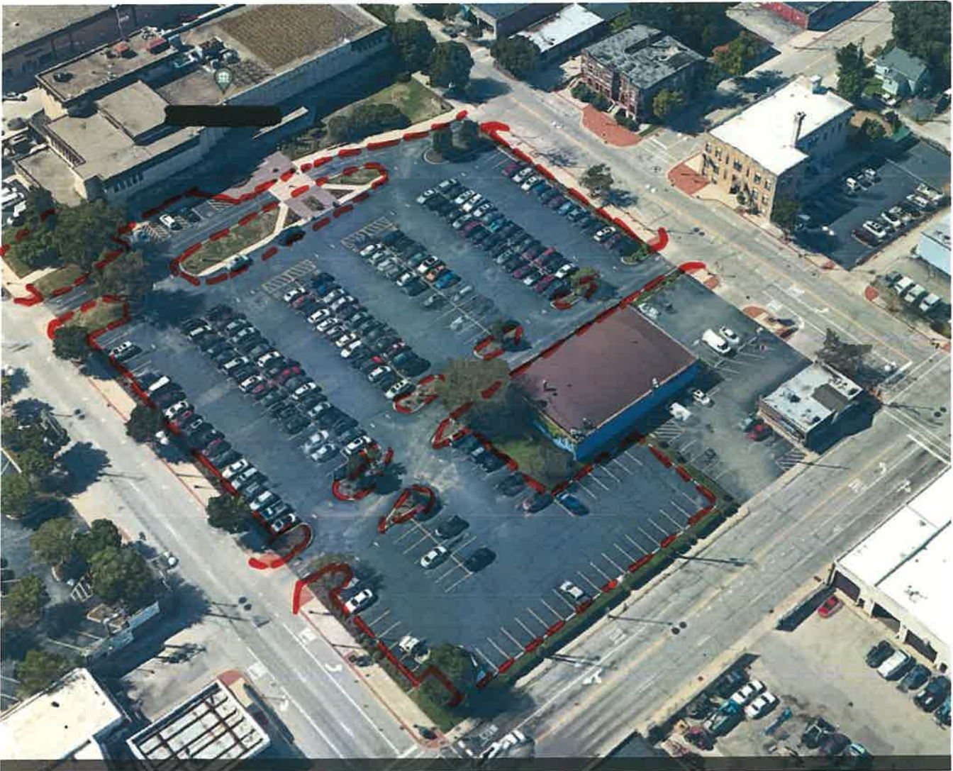
COUNTY OFFICE BUILDING
