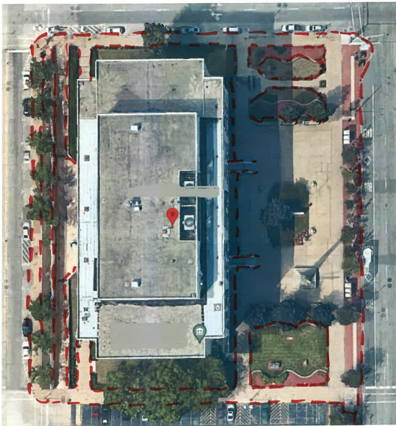
WILL COUNTY COURTYHOUSE (OLD)
